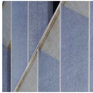
5. Precast Concrete Panels
