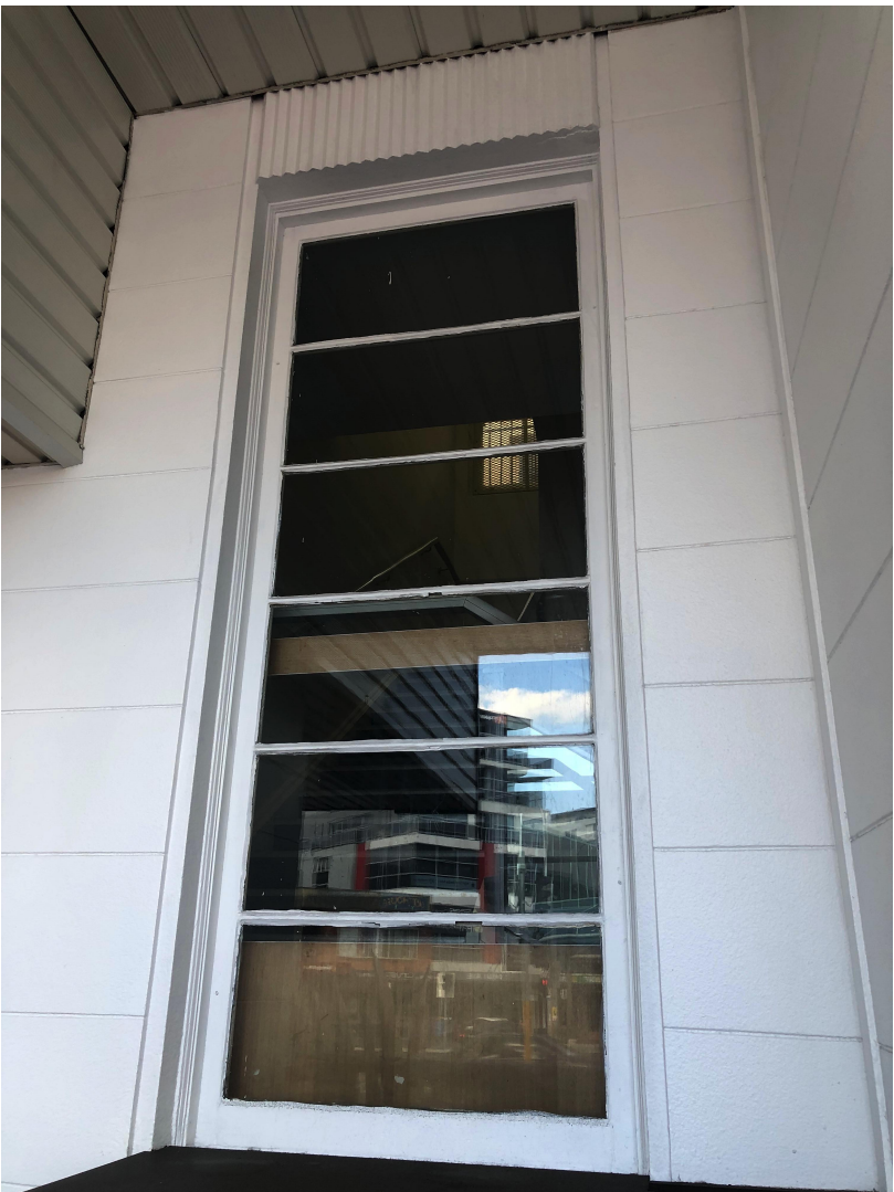
Window 1: Existing heritage window viewed from street, with staircase behind. Head detail to be matched in other restored window.
