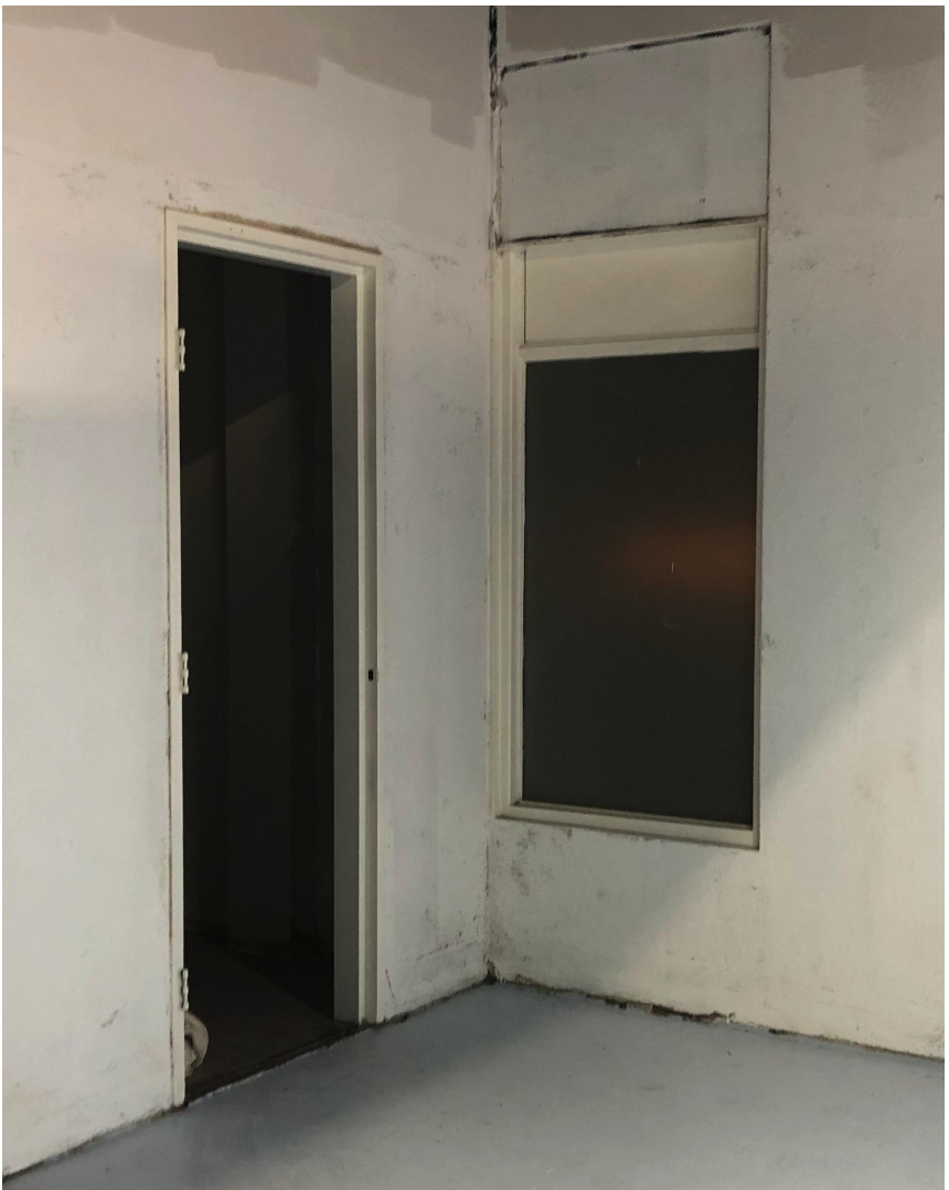
Window 2: Existing heritage window in poor condition. Currently covered by ATM services on the outside. View shown from inside existing building.
